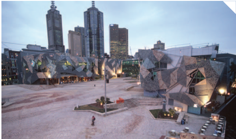
> FEDERATION SQUARE MELBOURNE AUSTRALIA PHOTOGRAPH COURTESY OF AWARD WINNING CONTRACTORS JA DODD LTD
